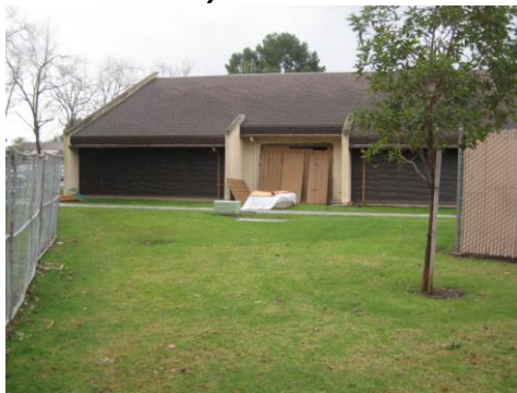
Removal of old siding
