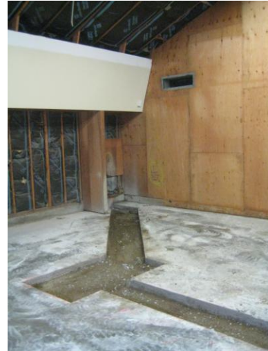
Plumbing the new science rooms...
