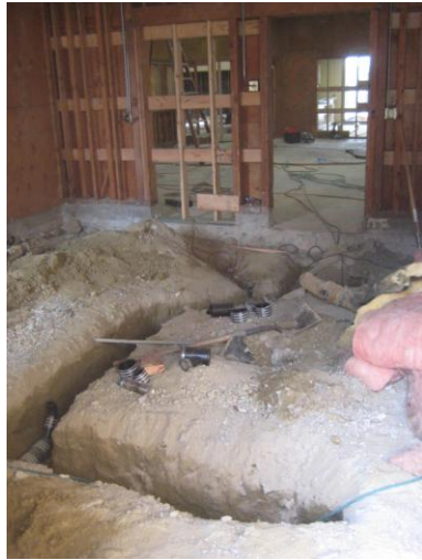
Laying pipe in the new bathrooms...
