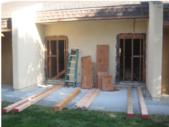
Breaking down the walls...
