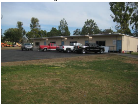
Our new asphalt area
