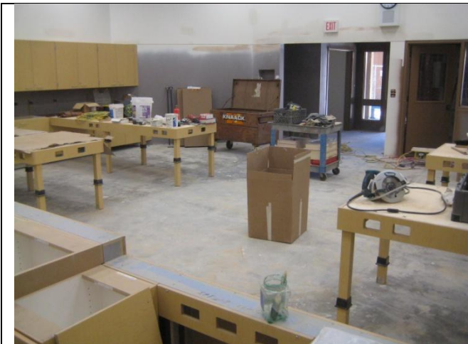
Installation of new tables & cabinets in science lab
