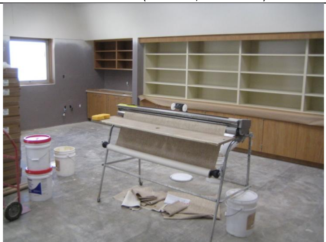
Wall papering of exterior rooms
