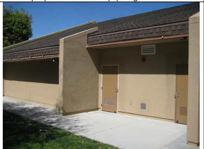
Exterior restroom paint & new doors
