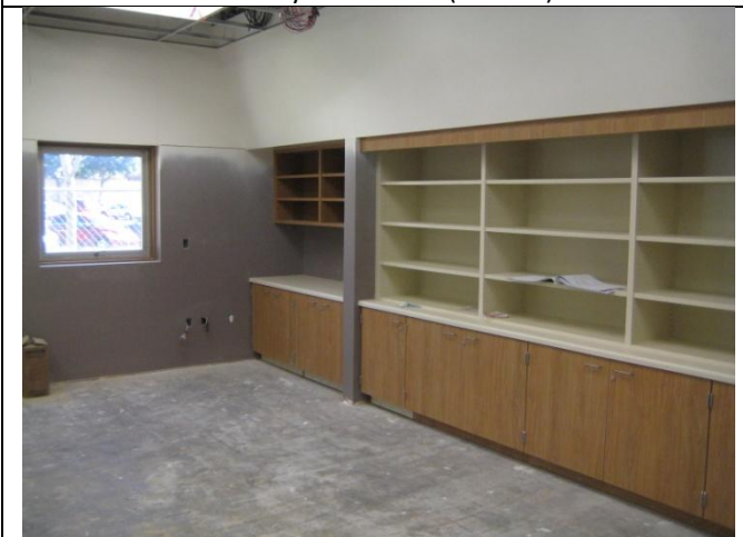
New cabinetry in exterior classrooms
